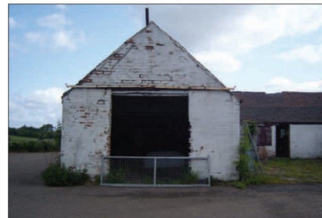
Southern elevation of the Forge viewed north east
