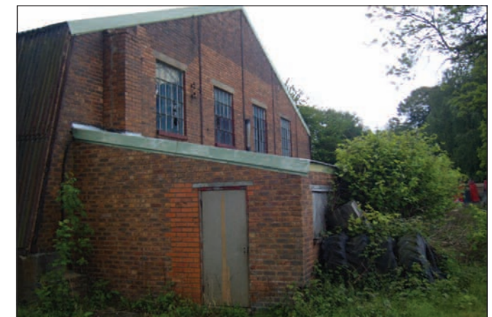
Southern elevation of the Central Garage Depot
