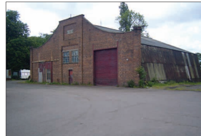
Front and western elevations of Central Garage Depot
