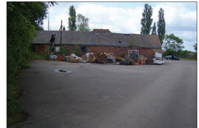
North elevation of the Forge viewed south west
