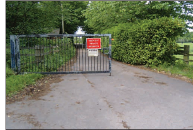
Vehicular access off Bursnips Road viewed west
